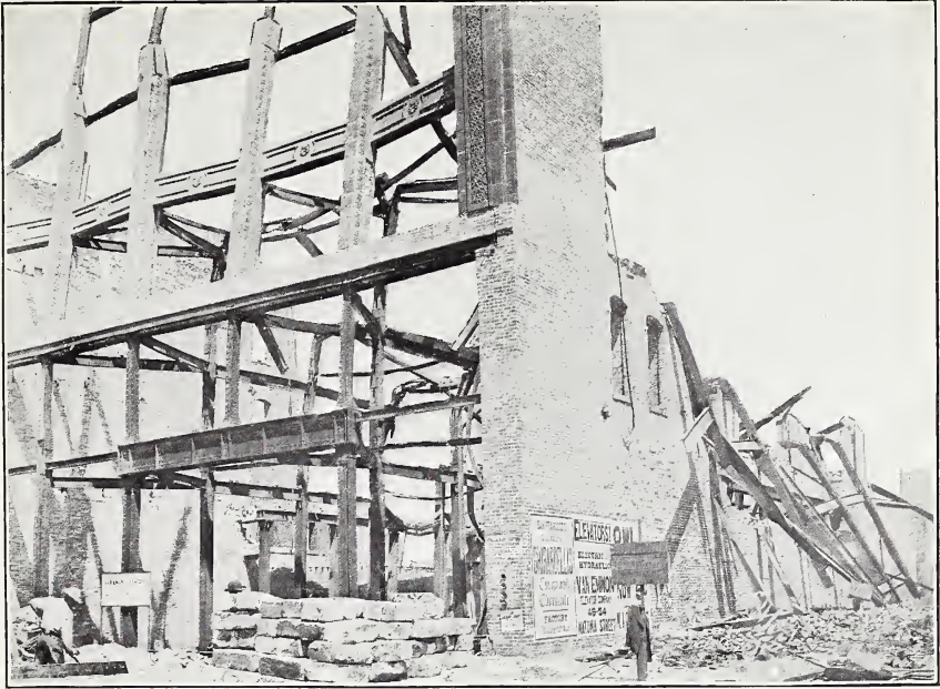
A. AN UNFINISHED STEEL SKELETON, WITH NONFIREPROOFED STEEL WORK.
